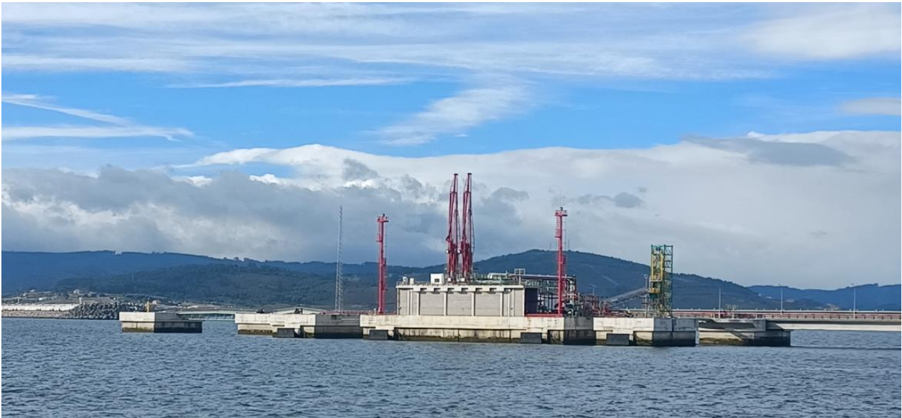
Figure 2. REPSOL pier at Punta Langosteira (Source: REPSOL)
